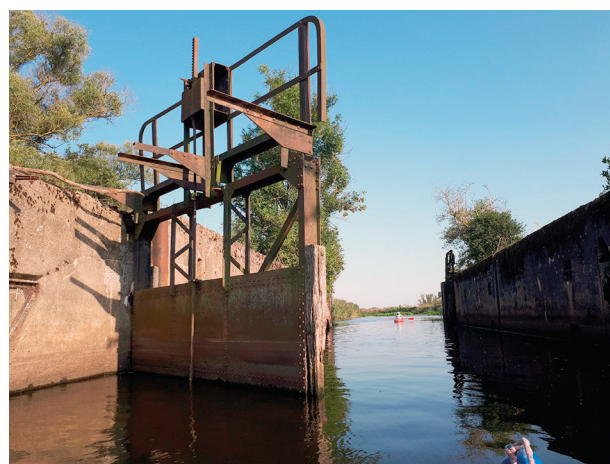
Figure 3. Unused lock in the Lower Oder Valley Landscape Park
